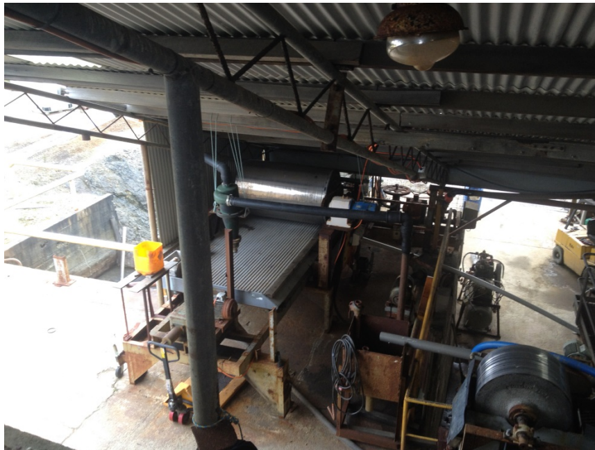
Figure 1: Section of the processing plant at the Granville Tin Project owned by ANW
