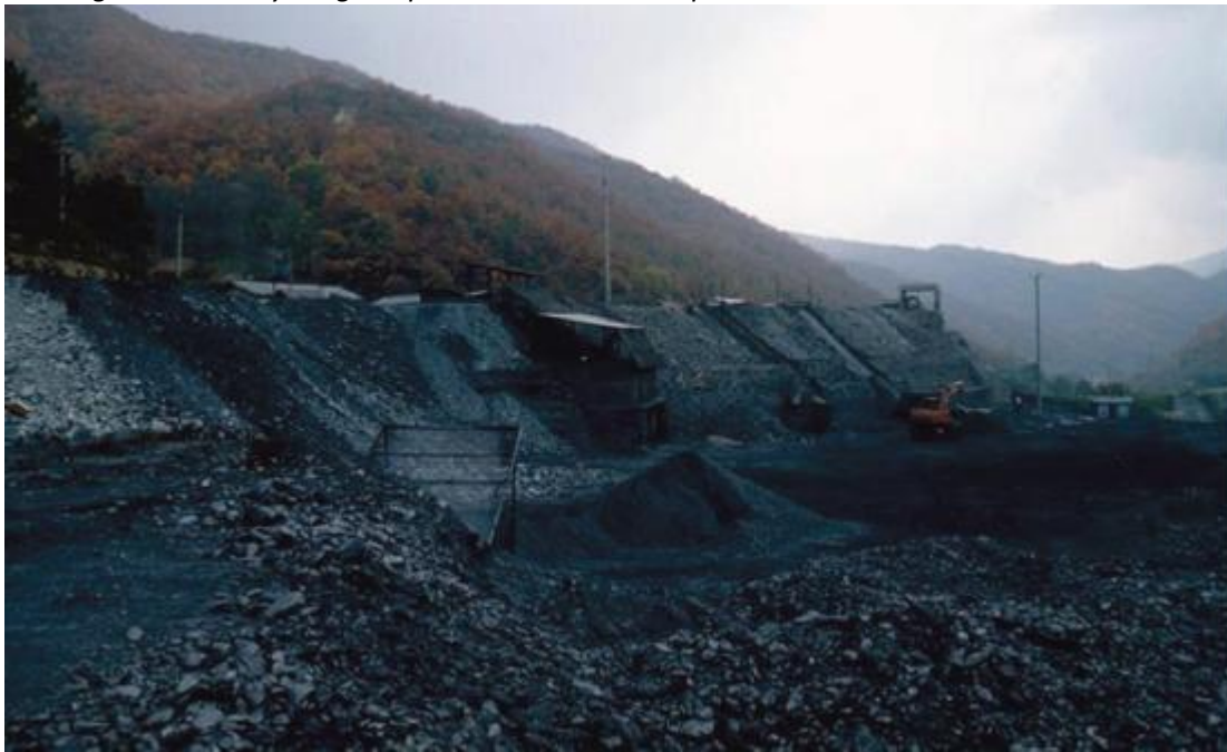
Figure 7: Wolmyeong Graphite Mine ROM Pad prior to the mine's closure in 1987 D8
