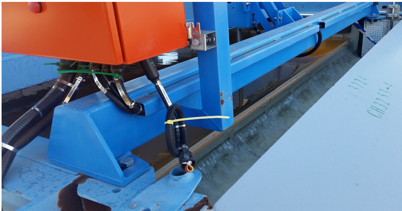
Figure 3: Wet commissioning of continuous gravity jigs.
