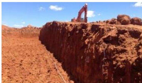
Figure 2: Good grade face of bauxite ore, Pit MB4
