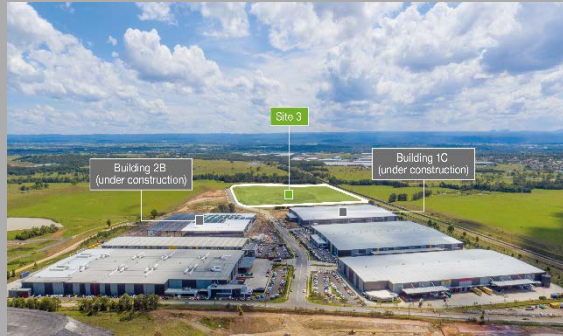
Oakdale Industrial Estate, Eastern Creek, Australia
