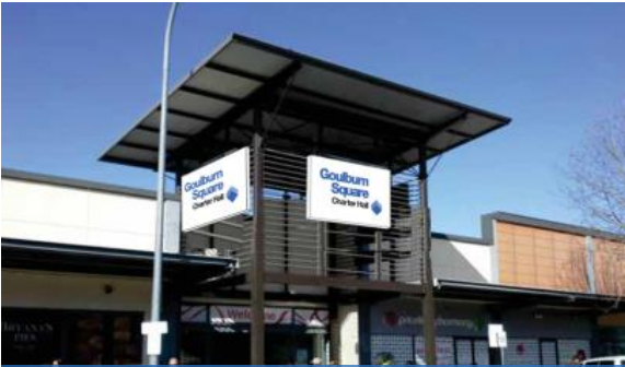
Goulburn Square, Goulburn (CQR)
