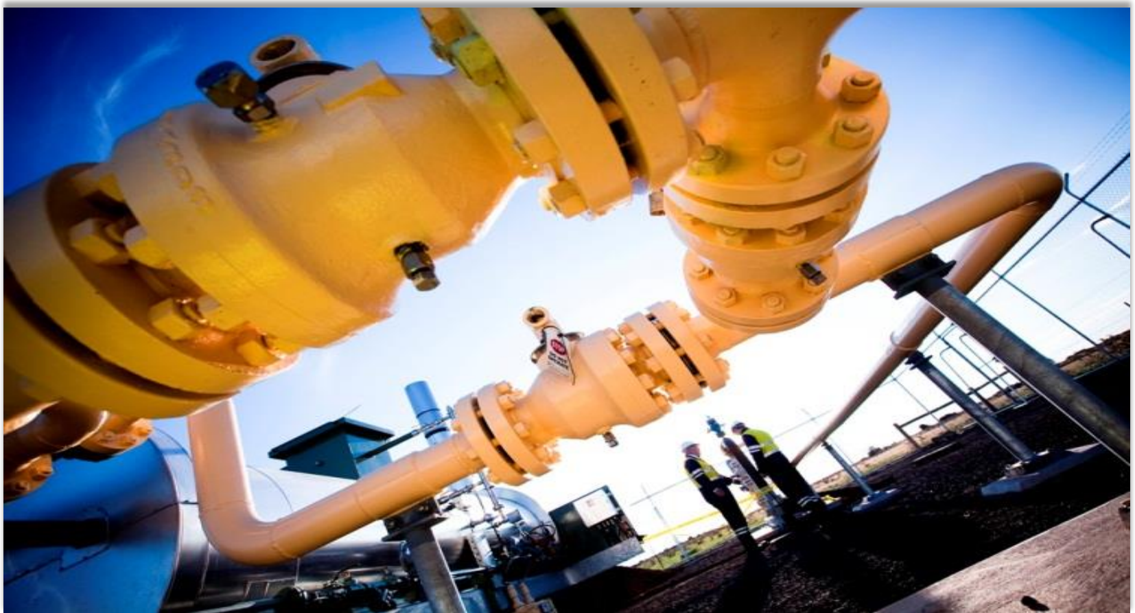
City gate pressure reduction asset
