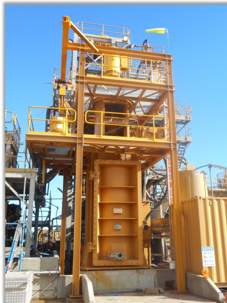
New Tower Mill – gravity circuit upgrade
