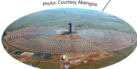
New Technology Delivery Khi Solar Tower, South Africa
