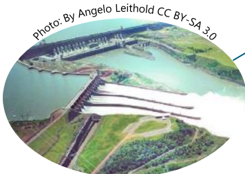
Mega Projects 14GW Repowering, Itaipu Project, Brazil
