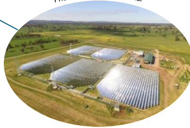
R&D Support Vast Solar Pilot Plant, Australia
