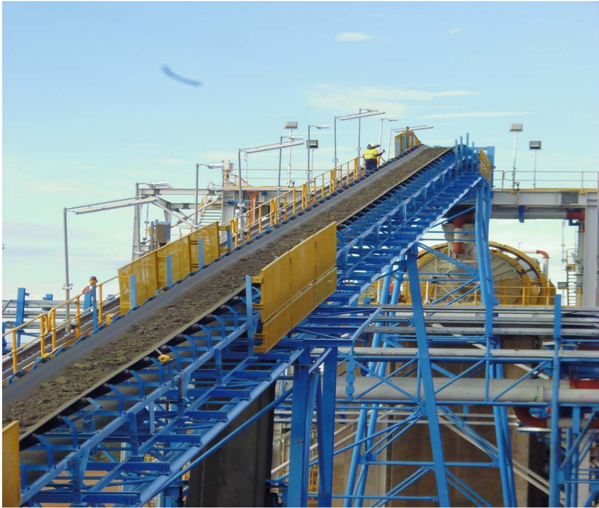
Ore feed going from the HPGR to the scrubber
