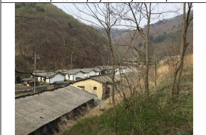
Abandoned Miners cottages and offices at Deuksu
