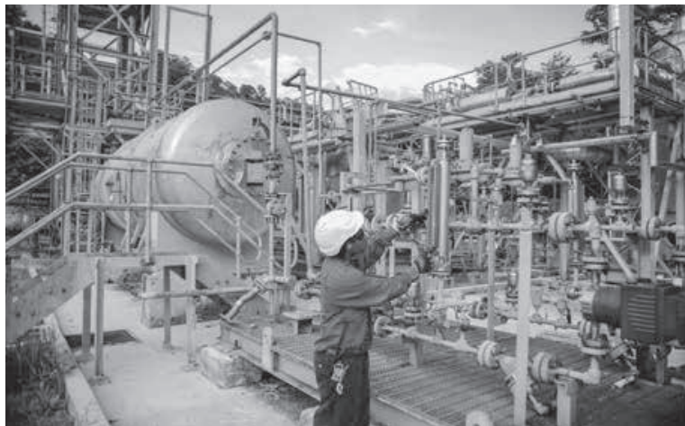
Central Processing Facility, Kutubu, PNG Highlands.
