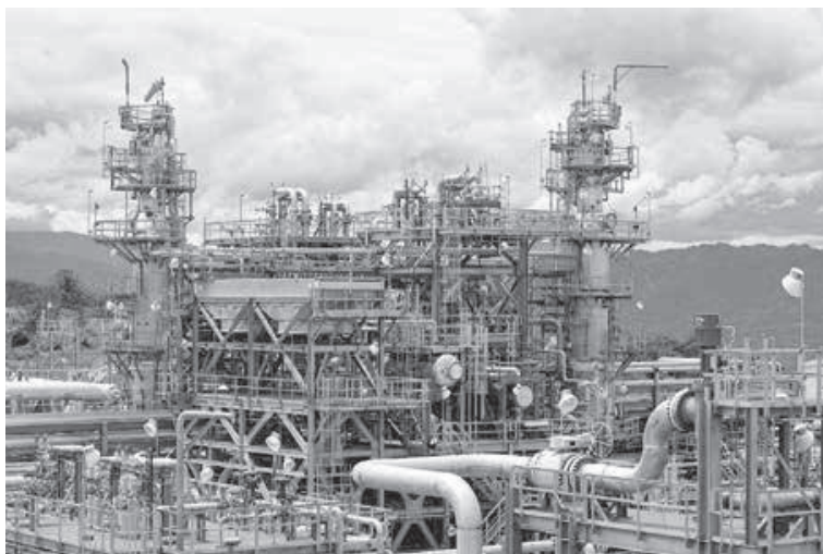
Hides Gas Conditioning Plant in the PNG Highlands. Photo courtesy of ExxonMobil.
