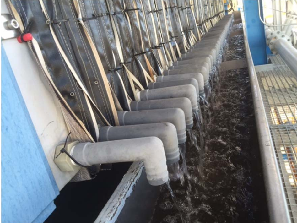
Filter plant in operation with water squeezed out
