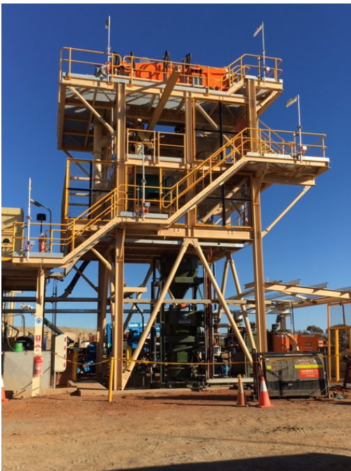
Figure 7 – Thunderbox mill - Gravity circuit installation
