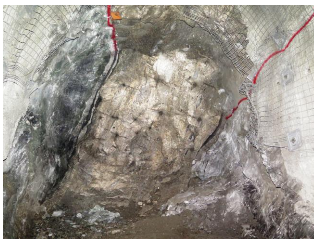
Massive ore in the 200 south ore drive with an average face grade of 5.0 % nickel
