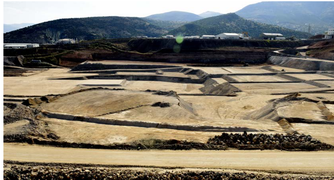
Sulfide Plant Site Earthworks Complete
