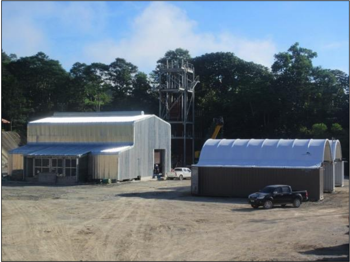
Photo 1: front left; winder house, front right; office and shop, back; headframe at 30%
