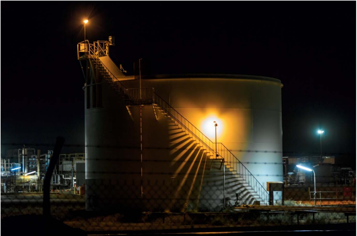
Figure 3: Mereenie; Crude oil tank at night.
