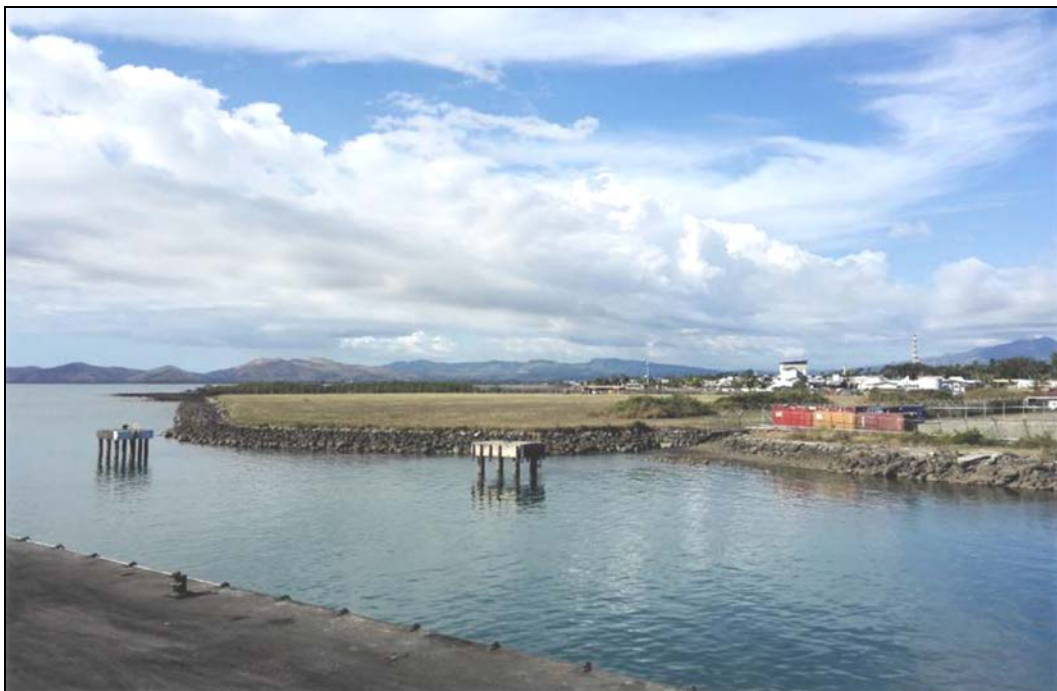
Amex Port Development Site, Lautoka
