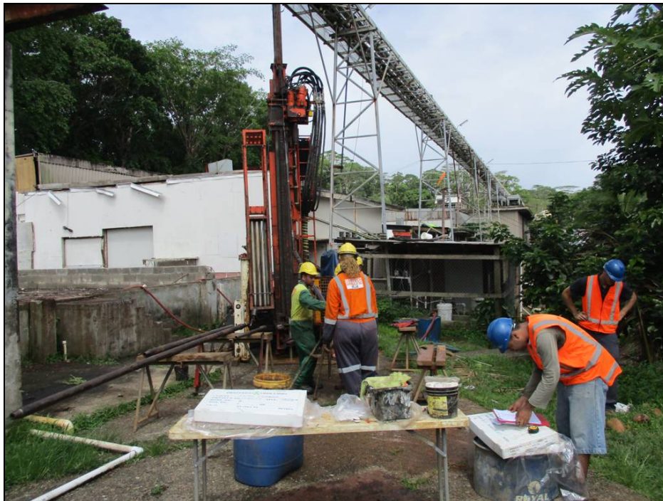
Geotech Drilling Operation, Fiji
