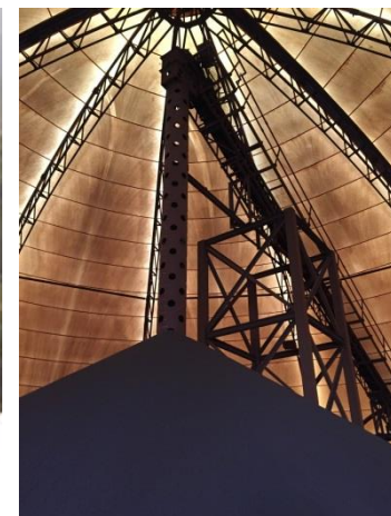
Rutile storage at Nitti Port
