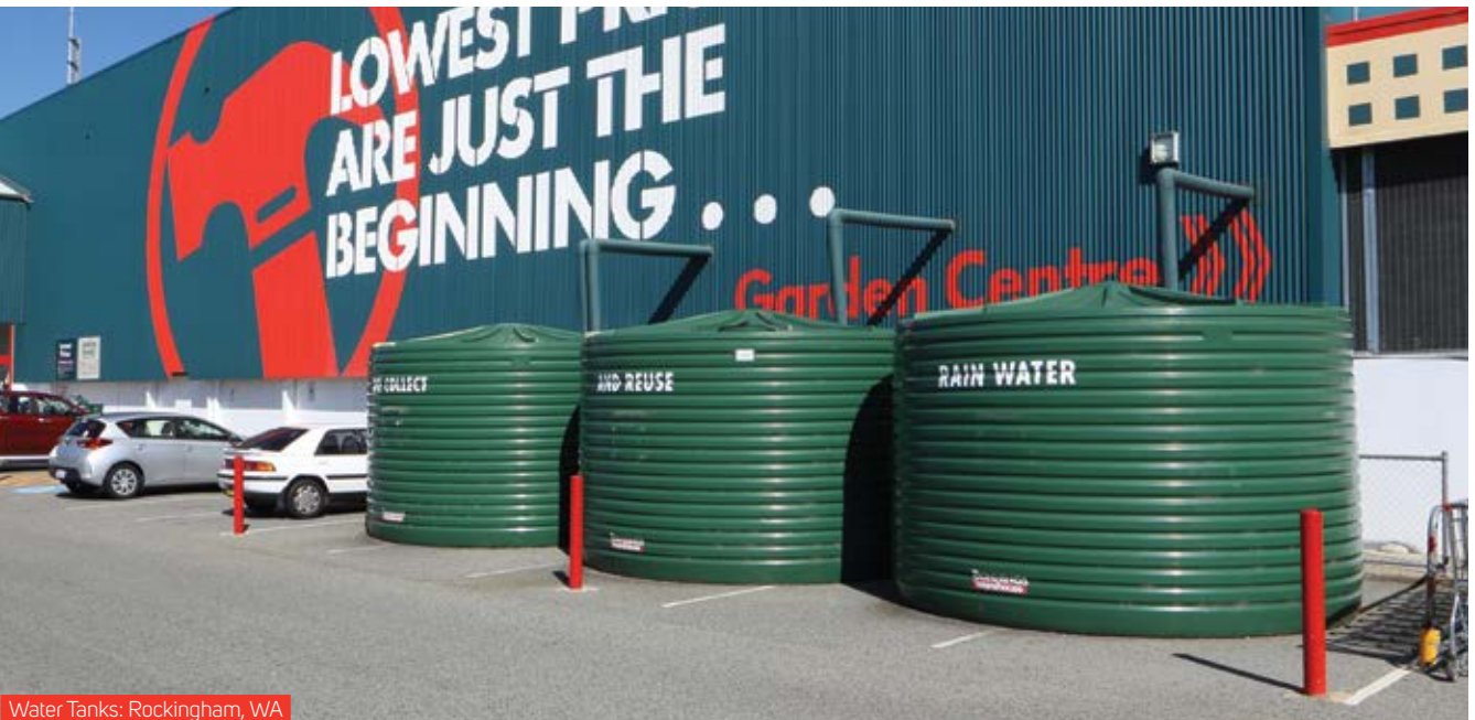
Water Tanks: Rockingham, WA
