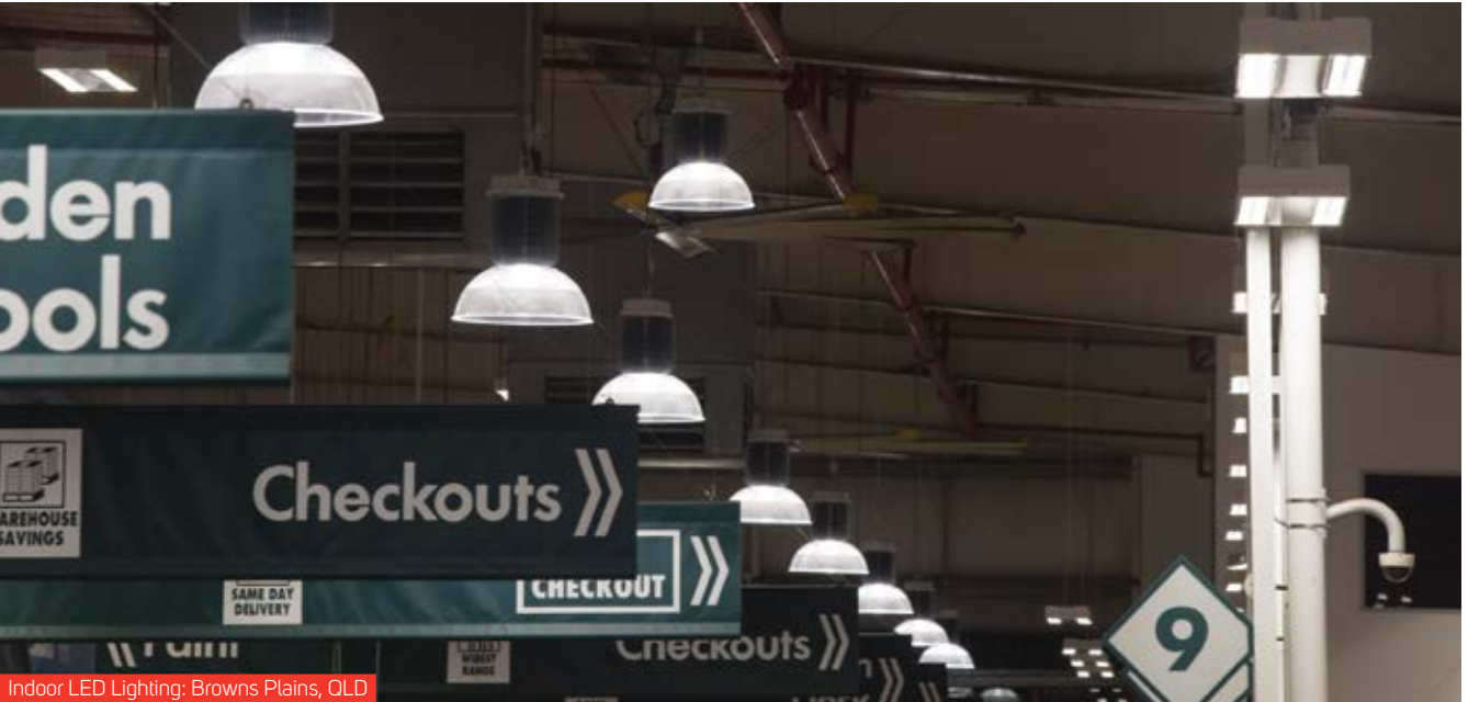
Indoor LED Lighting: Browns Plains, QLD
