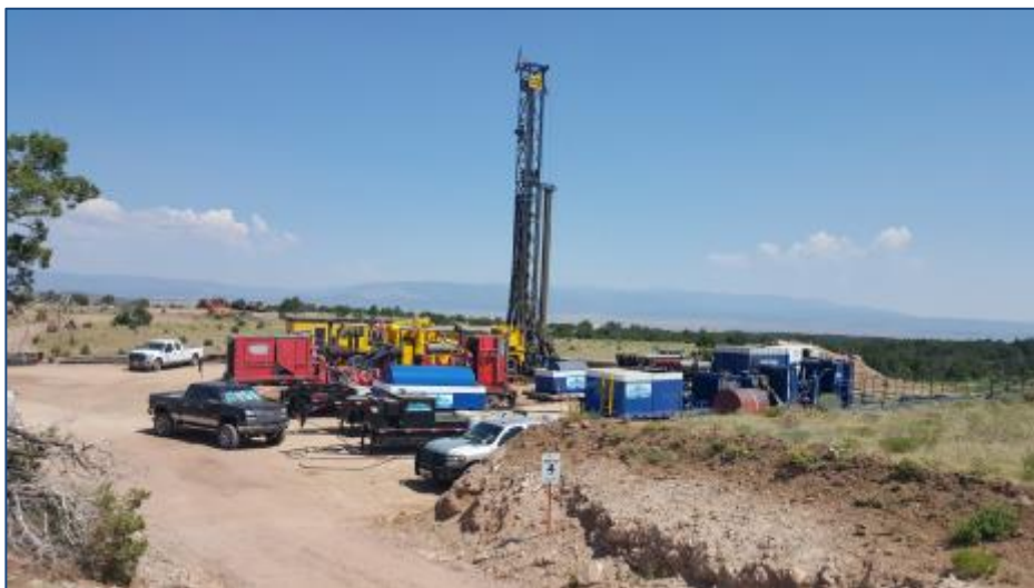
Drilling Operations Underway on the Marco Polo #1 well targeting oil production from the Pierre Shale Formation
