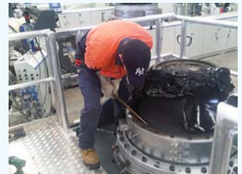
THE HEIGHT OF THE PLATFORM MEANS THAT OPERATORS CAN WORK AT THE SAME LEVEL AS THE TOOLING MACHINE.
