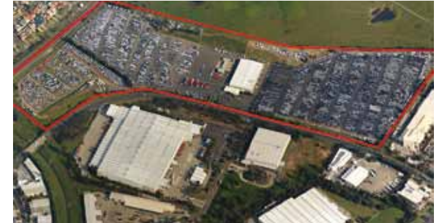
Ingleburn Distribution Centre
