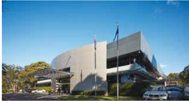
Macquarie Technology Centre
