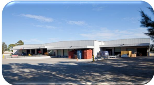
457 WATERLOO ROAD, CHULLORA NSW
