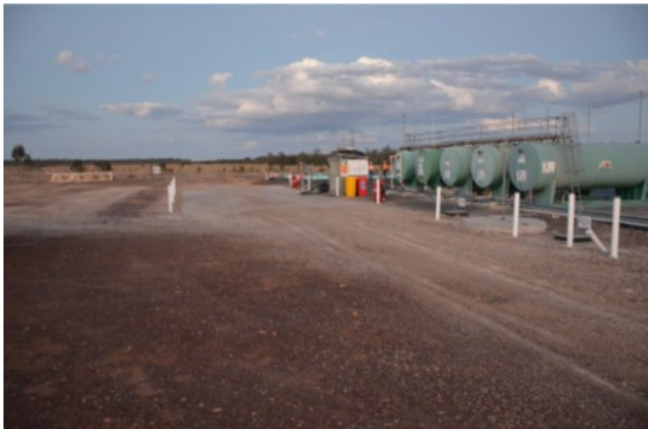
Figure 2: Emu Apple facility including offloading area
