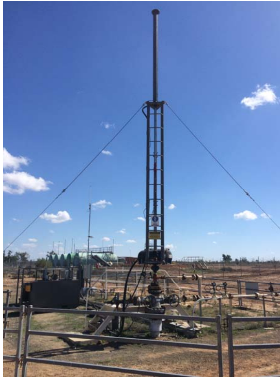
Figure 1: Emu Apple-1 well with storage tanks in the background
