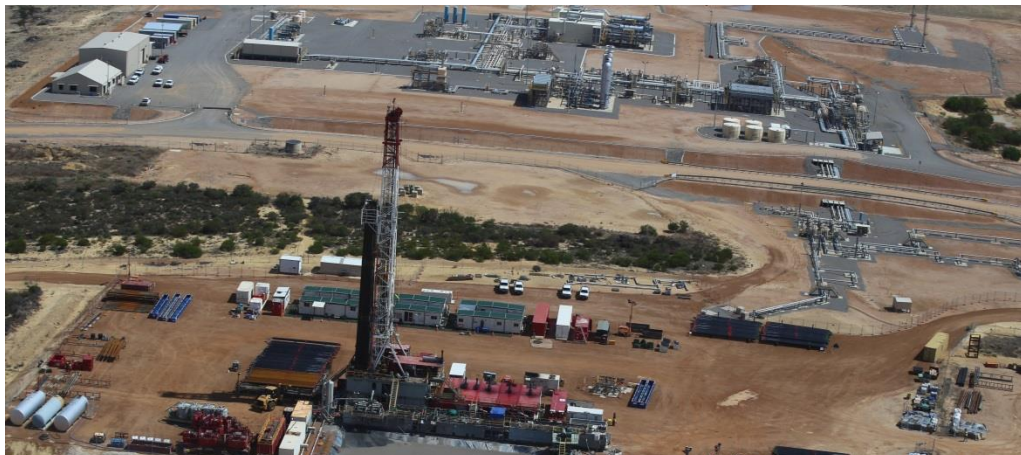
New injection and withdrawal well completed at Mondarra Gas Storage Facility during FY16, increasing storage
