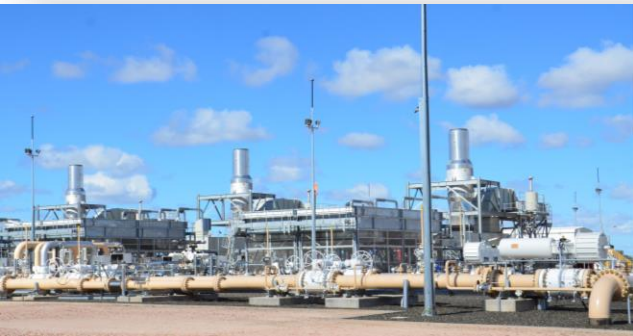
Wallumbilla Compressor Station
