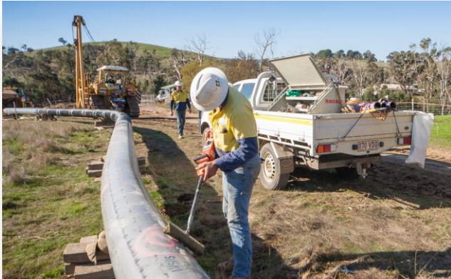
VNI expansion works
