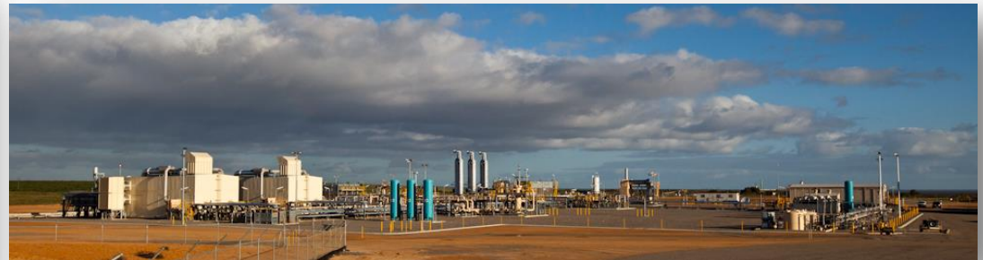
Mondarra Gas Storage Facility
