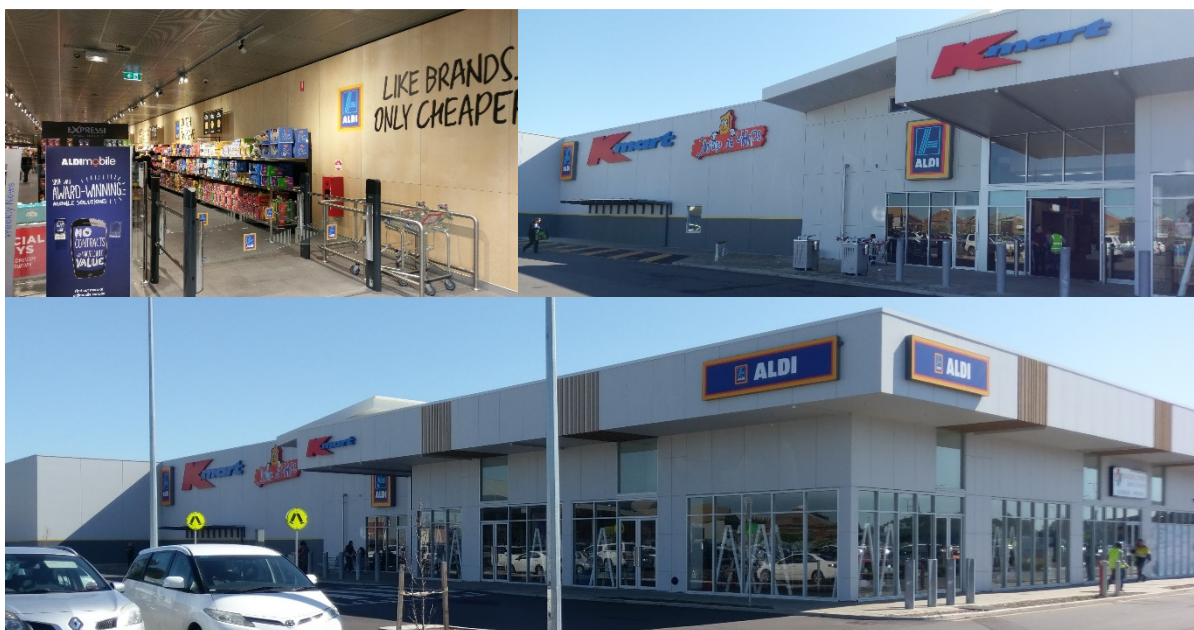
Churchill Centre North Aldi extension
