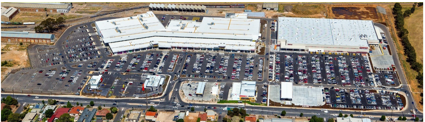
Churchill Centre North
