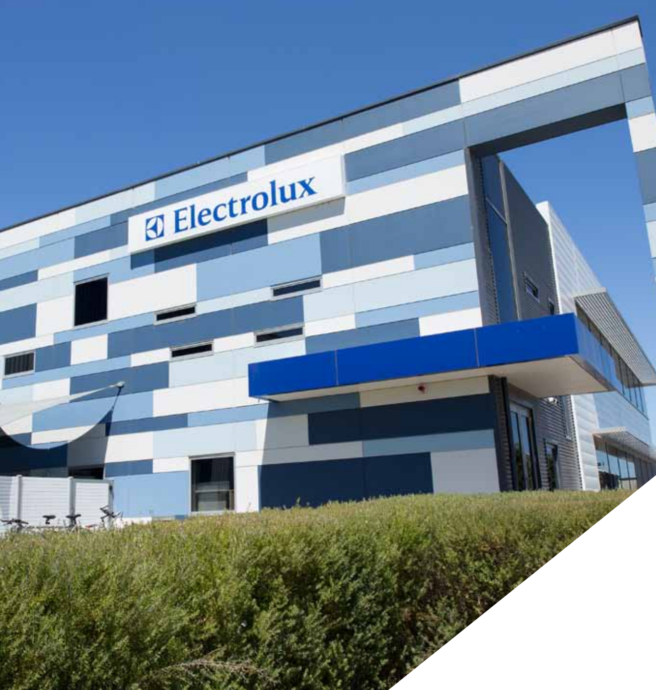
Electrolux Distribution Centre, 76-80 Howards Road, Beverly SA
