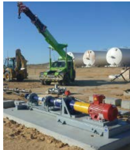
Construction of Pennington facility in ex PEL 91
