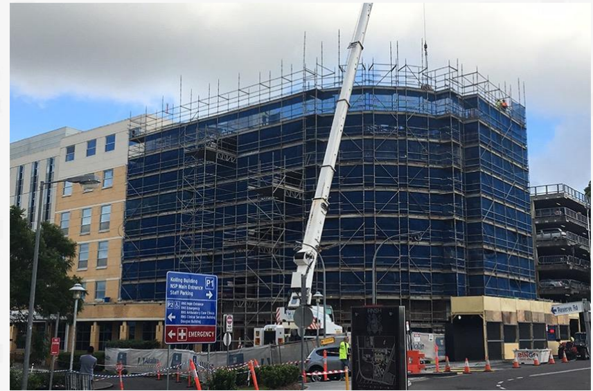
North Shore Private Hospital extension under construction
