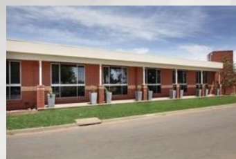
Shepparton Private Hospital (new mental health and rehabilitation wing)
