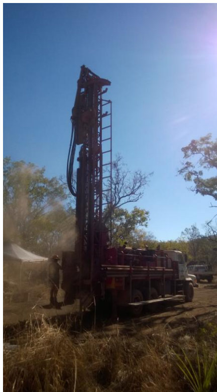
Figure 2 Drill rig on site at Mt Porter drilling Water Monitoring Bores
