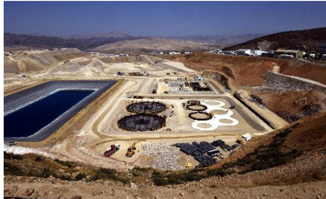
Sulfide Plant Expansion Progress
