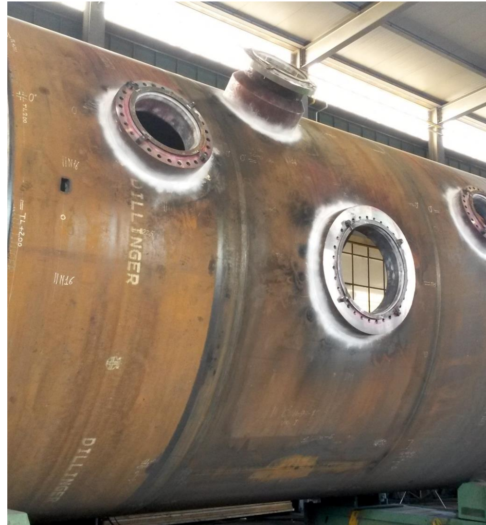
Çöpler autoclave shell in fabrication
