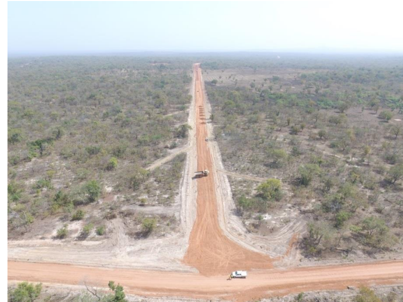
Left: Sissingué access road works underway
