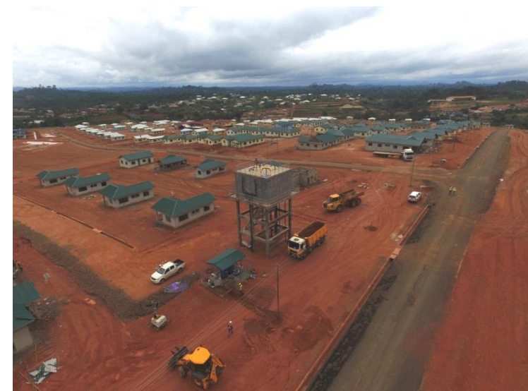
Bottom Left: General view of water tower and housing estate
