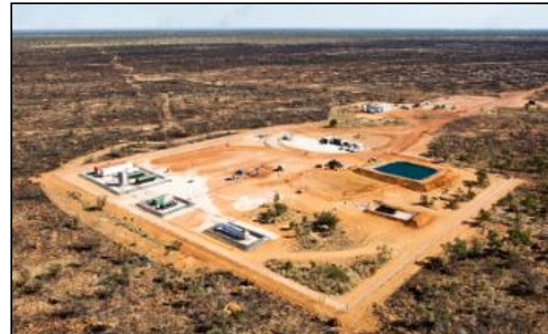
Ungani field facility
