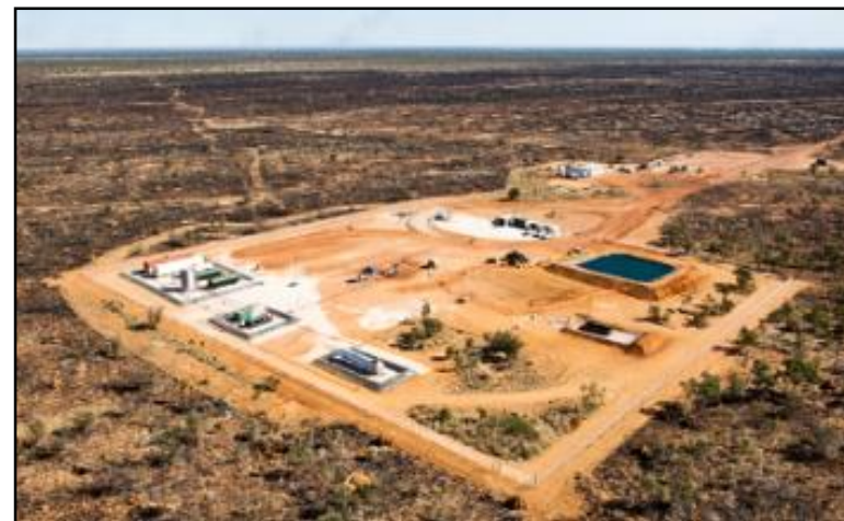
Ungani field facility
