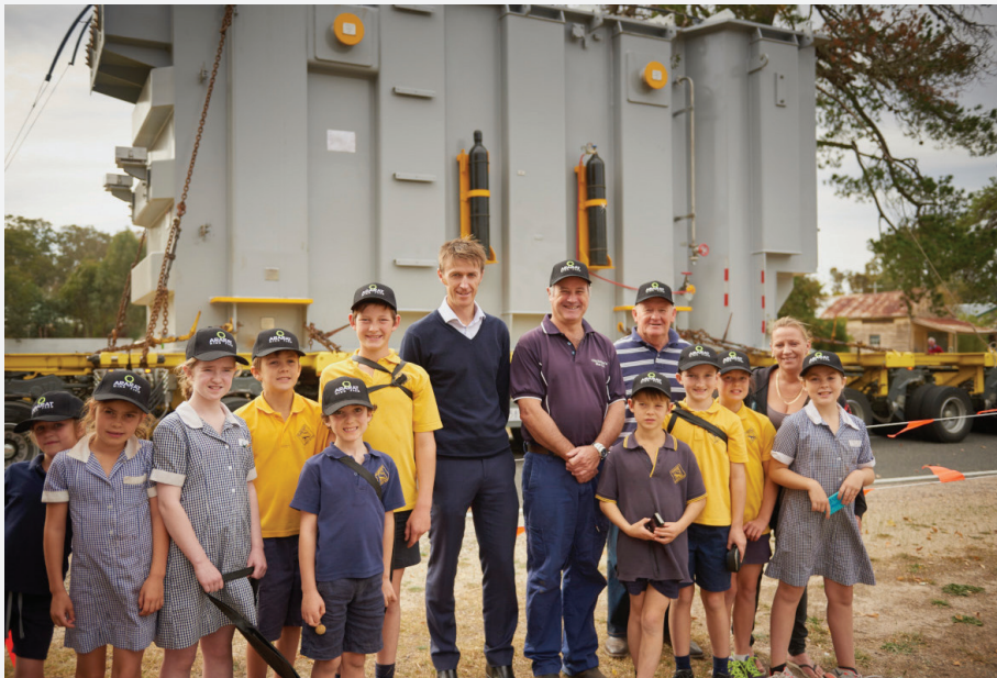
TRANSFORMER ARRIVES AT ARARAT TERMINAL STATION
