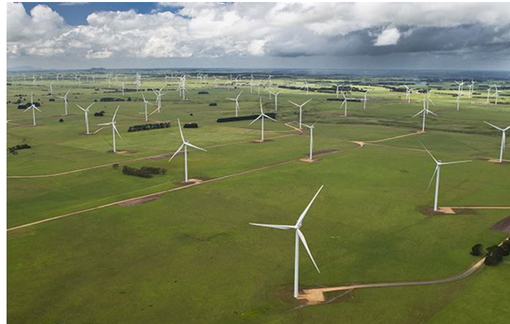
Macarthur Wind Farm: AusNet Services built the terminal station to connect 420MW wind farm near Tarrone, Victoria.
