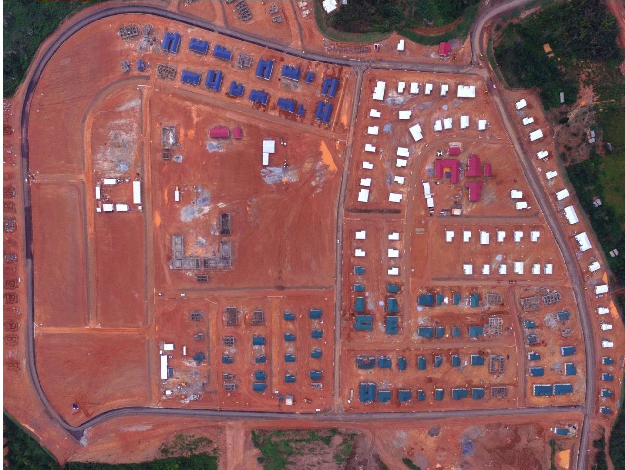
Above: Aerial view of relocation housing estate
