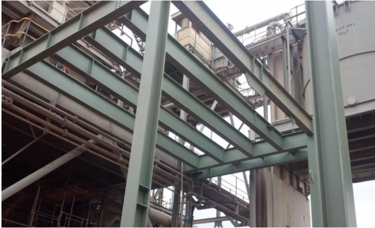
Above: Steelwork for expansion of SAG Mill floor to facilitate efficient mill relines
