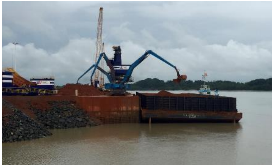
WAP barge load-out facility at Katougouma, Guinea (August 2016)
