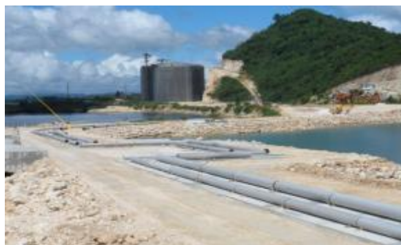
Stainless Steel Pipeline
