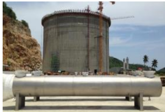
Installation of Regasification Unit
