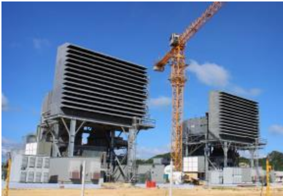
Construction of Power Plant
