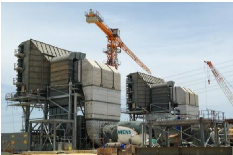
Pagbilao Power Plant
