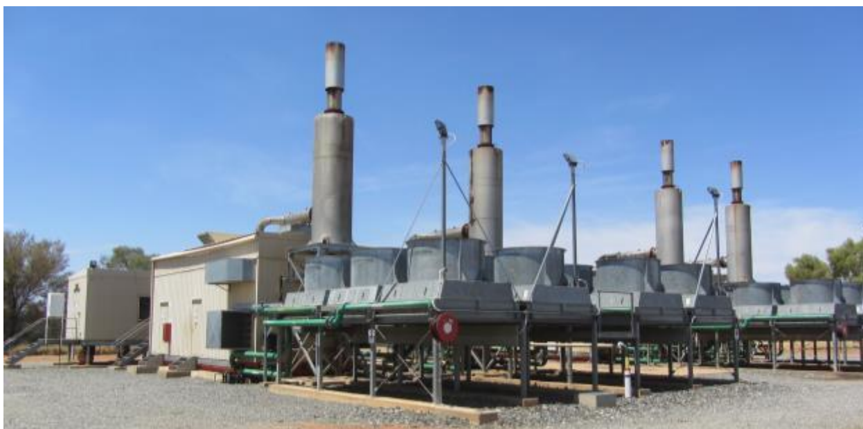
Alice Springs Power Plant, Australia
