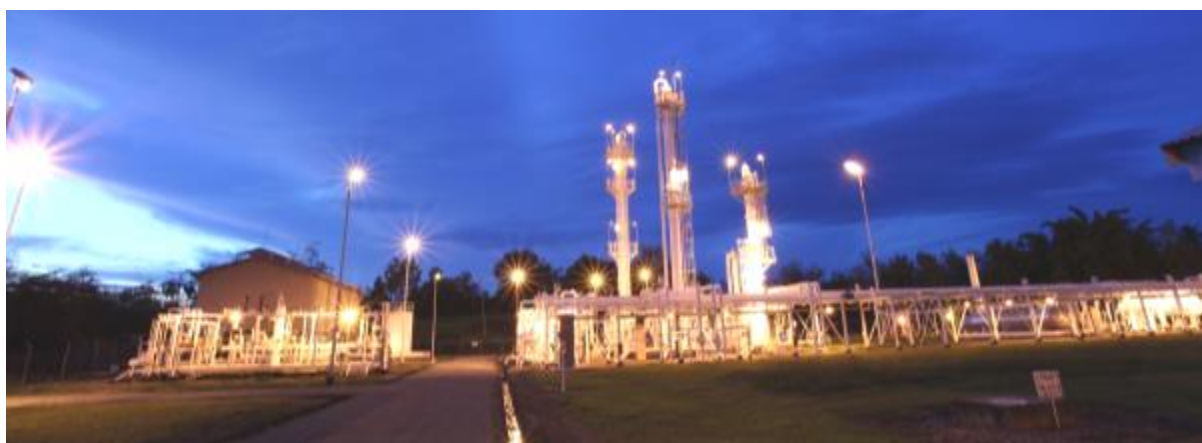
EEES Kampung Baru Sengkang, Indonesia Central Processing Plant (CPP)
