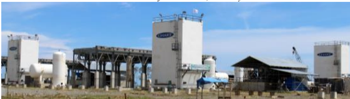
Main Processing Plant Area
