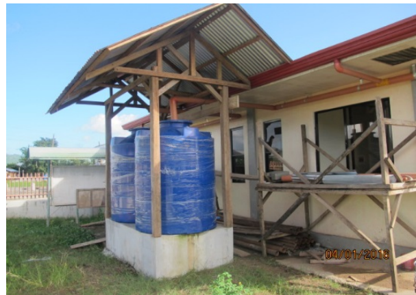
Photo: Rain water tank installed
