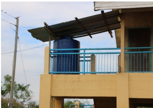
Photo: Rain water tank installed
