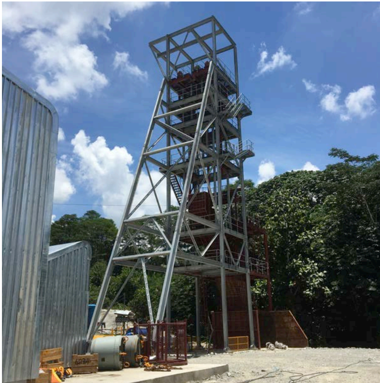
Picture 3 E15 Head Frame at 80% completion
