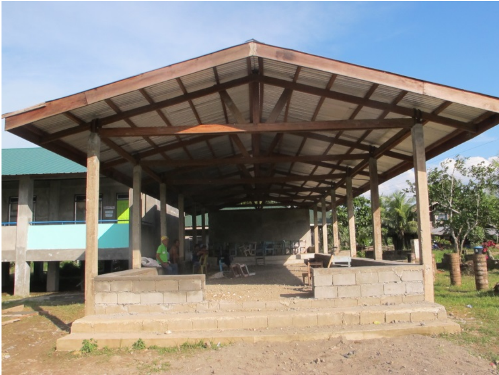
Photo: Newly constructed Social Hall at existing premises of school
