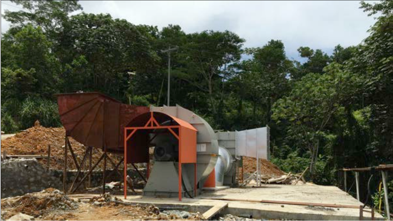
Picture 5. The 2 new Centrifugal Fans before commissioning
