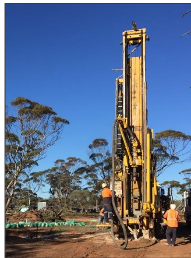
Current Paris infill RC drilling
