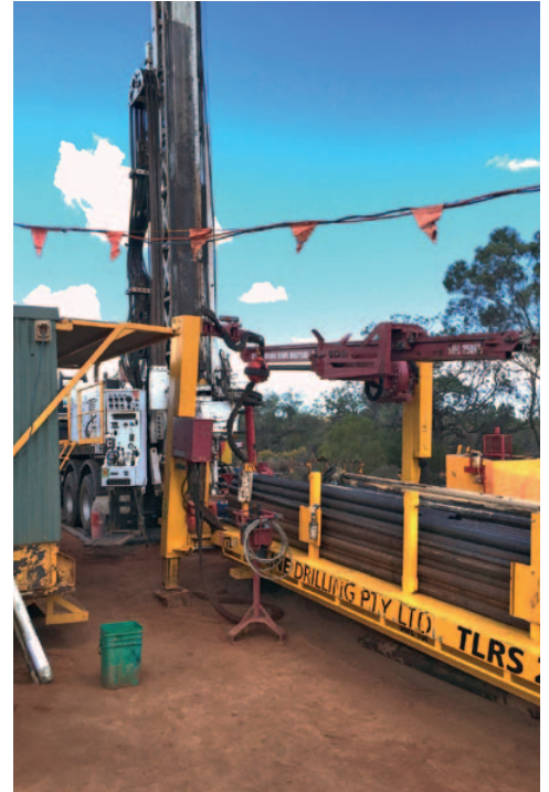
Drilling first Nankivel diamond hole, August 2016.
