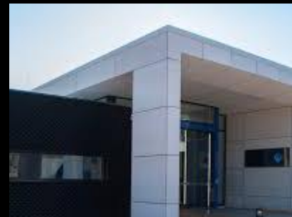
Intellicentre 4 Bunker, Canberra
