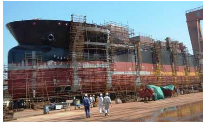
New ship during construction
