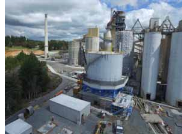
New Silo under construction (foreground) at manufacturing plant, Whangarei
