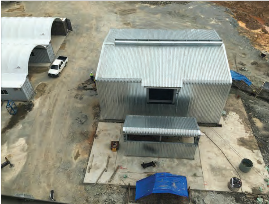
Picture 4: Winder House (centre) and Offices (left) from top of Head Frame
