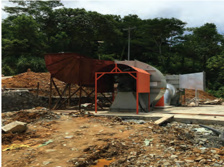
Picture 5: The 2 new Centrifugal Fans before commissioning
