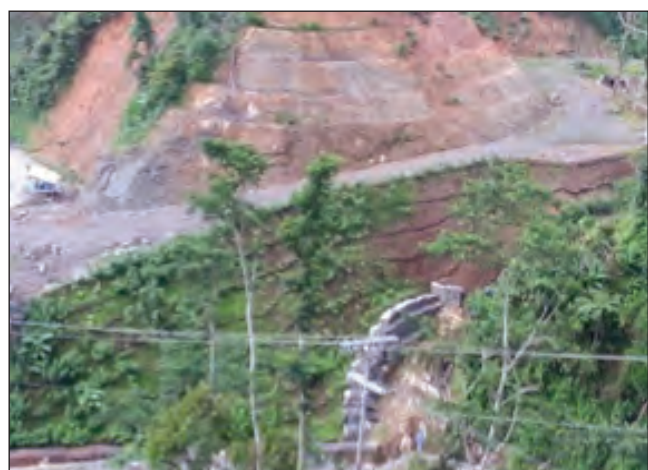
Photo: Revegetation on Slopes
