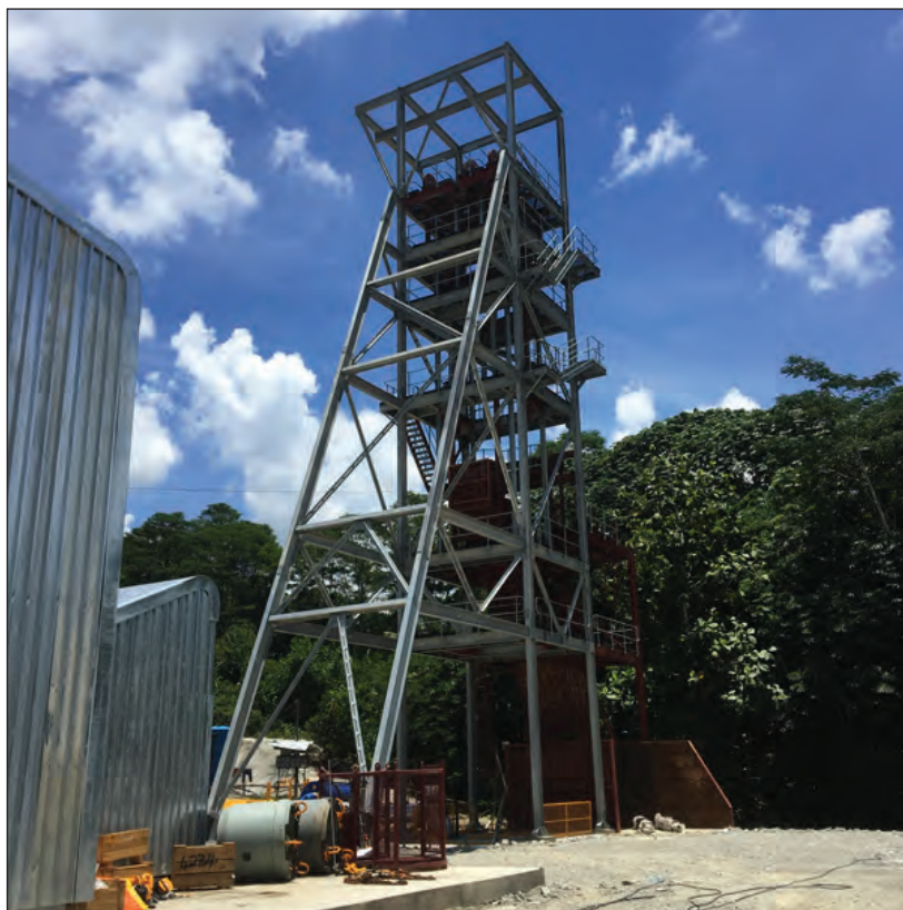
Picture 3: E15 Head Frame at 80% completion
