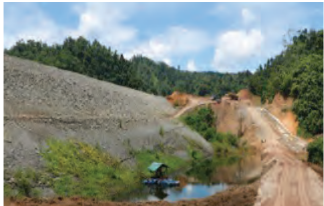
Picture 2: shows tails storage facility #5 downstream of main dam showing freshwater spillway still under construction
