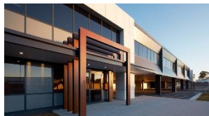
Ingleburn Distribution Centre, NSW
