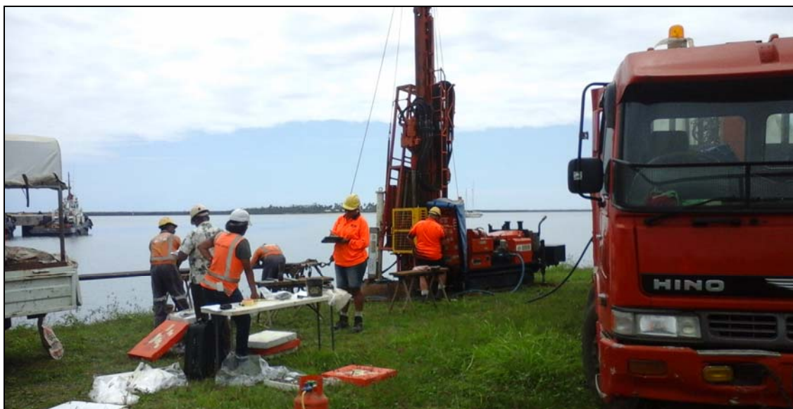
Geotechnical Drilling Amex Lautoka Port
